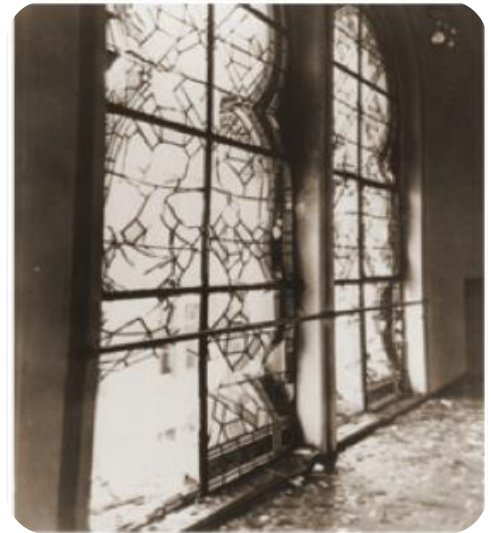
The shattered stained-glass windows of the Zerrennerstrasse synagogue after its destruction on Kristallnacht. Pforzheim, Germany, ca. November 10, 1938.
